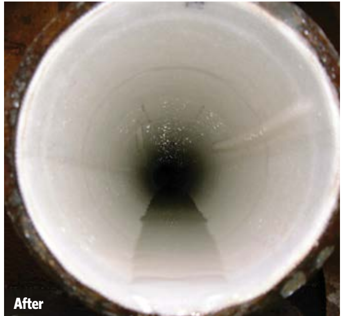
Epoxy migrates through the outer jacket of the liner to fill all voids around the services and any existing spaces within the host pipe, creating a full bond to the interior of the old water main
